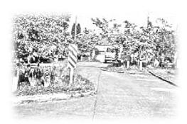
Chicanes are curb extensions that alternate from one side of the street to the other, forming S-shaped curves. Chicanes can also be created by alternating on street parking, either diagonally or parallel, between one side of the street and the other. Each parking bay can be created either by restriping the roadway or by installing raised landscaping islands at the end of each parking bay.
