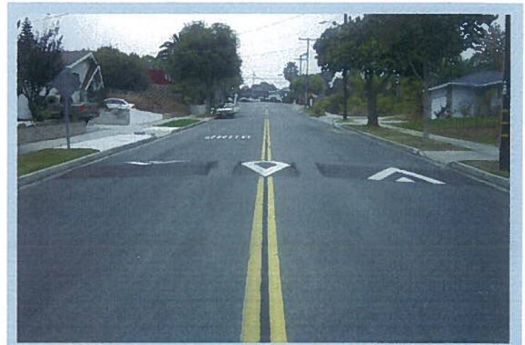
Carey Road, Oceanside
